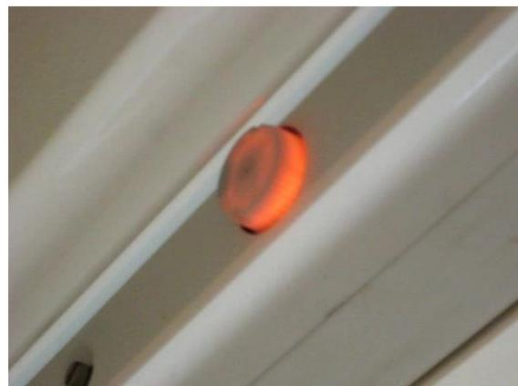
Starting a preheat lamp. The automatic starter switch flashes orange each time it attempts to start the lamp.
